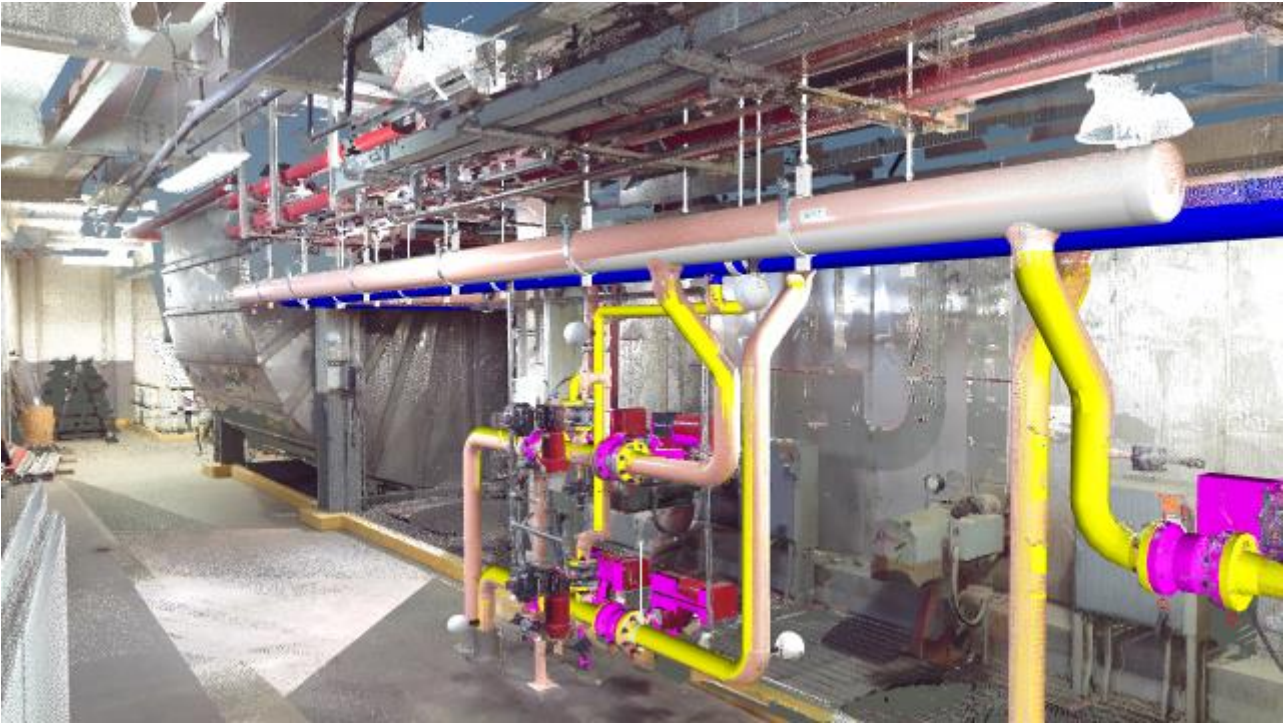
3D Laser Point Cloud Data Conversion to Intelligent 3D Model
